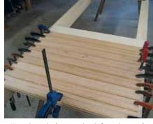
2. Using the poplar frame as a handy flat and true surface, the next step is to glue together the truck's dashboard out of traditional tongue-and-groove red oak bead board.
